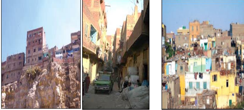
Figure (4): Features of Nasser's deteriorating facility [13]
