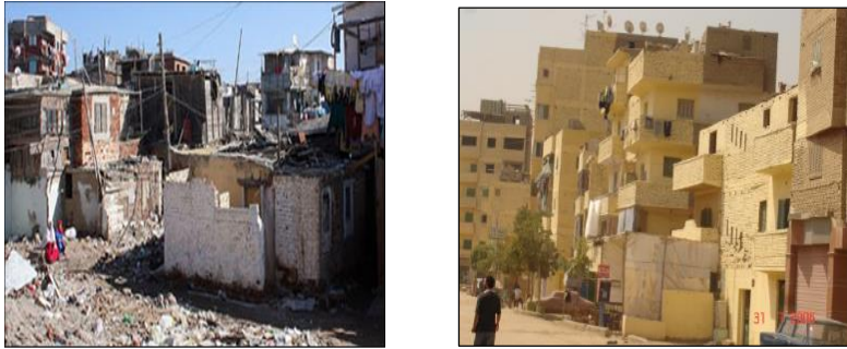
Figure (3): Izbet Al-Walda area before & after the development [9]
